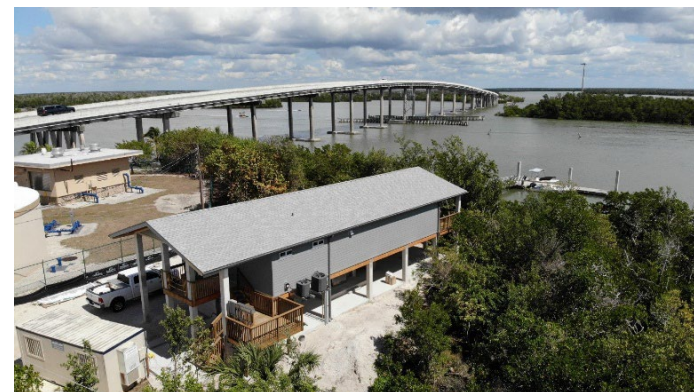
The Goodland Field Station at the Rookery Bay NERR provides dormitory space for students and visiting scientists
